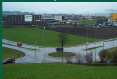
A recent Swiss scheme replacing signals
