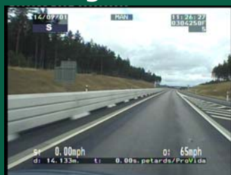
Central safety fences on single carriageways - now the Swedish standard
